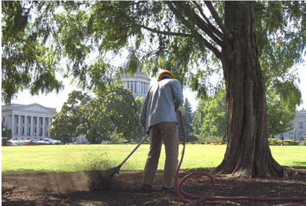
Figure 3. An Air Spade or Vertical Mulching Can Decompact Soils
